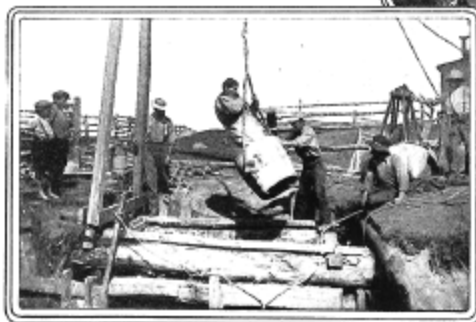
The diver entering the pit
